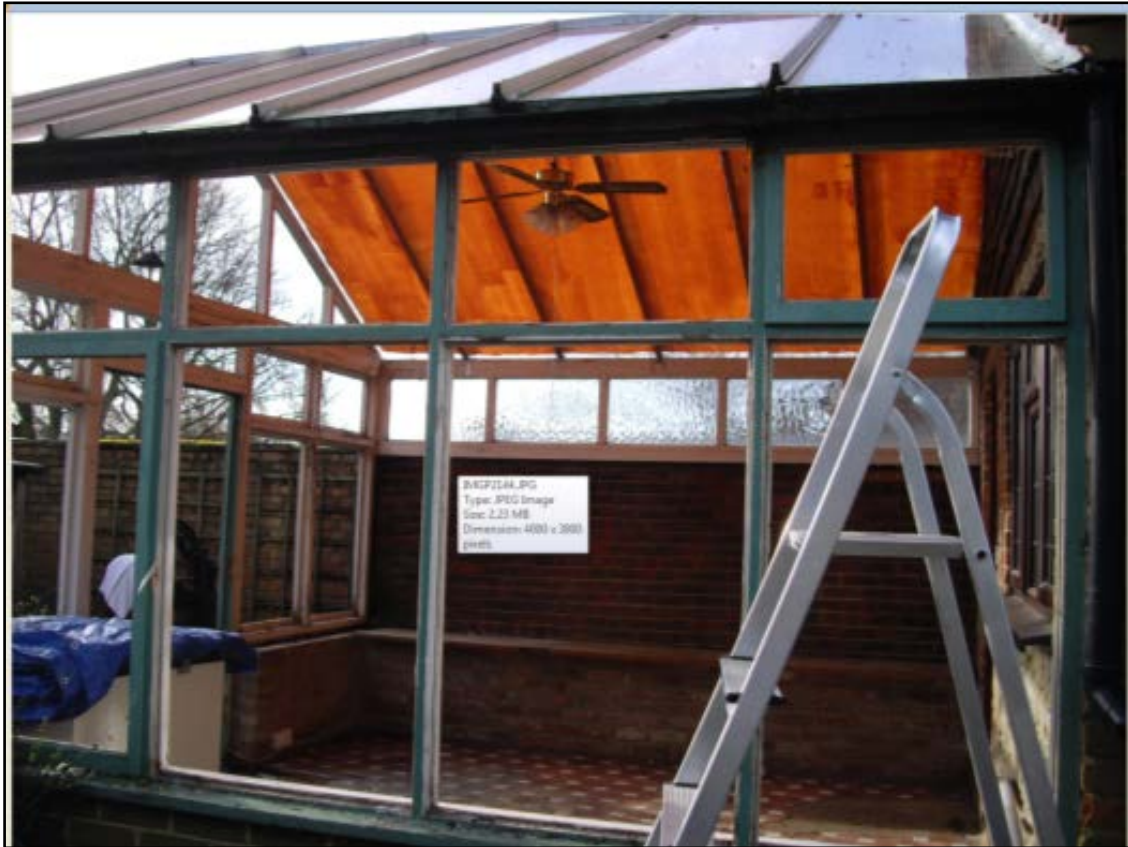
Figure 8. Picture of building/conservatory prior to rebuild works showing the high level windows on the side (NW) elevation facing the neighbour.
